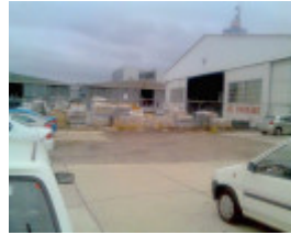
H0094 CAC hangars 2006
