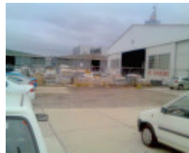
H0094 CAC hangars 2006
