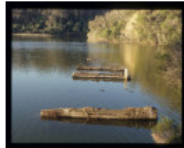
LAKE TYERS TIMBER COMPANY TRAMWAY BRIDGE
