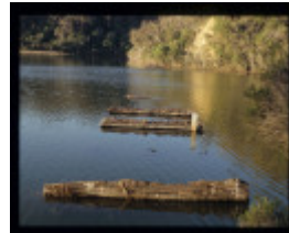
LAKE TYERS TIMBER COMPANY TRAMWAY BRIDGE
