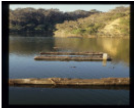
LAKE TYERS TIMBER COMPANY TRAMWAY BRIDGE
