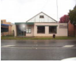
Rsl Hall & Flagpole, former
