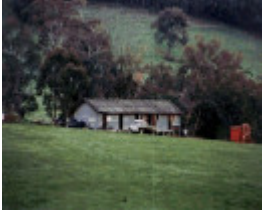
Former army hut
