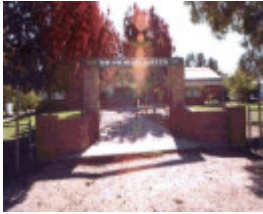
Chiltern Primary School Memorial Gates
