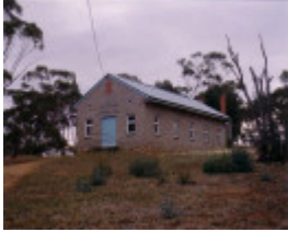
SC 01 - Shire of Northern Grampians - Stage 2 Heritage Study, 2004
