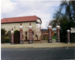
SL 167 - Central Park, including Memorials and Ticket Booths, Main Street, STAWELL
