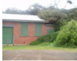
Powder Store, Point Lonsdale Road, Queenscliff
