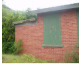
Powder Store, Point Lonsdale Road, Queenscliff
