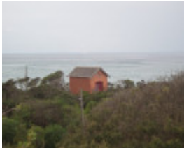
Powder Store, Point Lonsdale Road, Queenscliff
