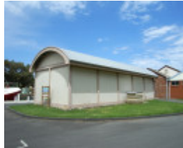
FORMER CUSTOMS SHED SOHE 2008
