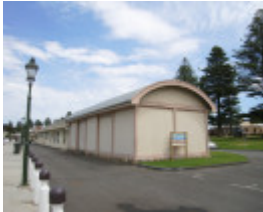
FORMER CUSTOMS SHED SOHE 2008
