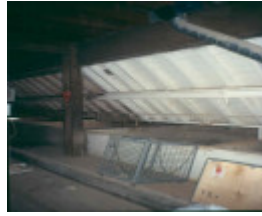
h02050 richmond maltings steeps and grain hoppers 1930 malthouse mz june03
