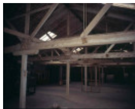
h02050 richmond maltings first floor 1920 malthouse mz june03
