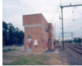
h02025 1 bunyip sub stationjul03 jc
