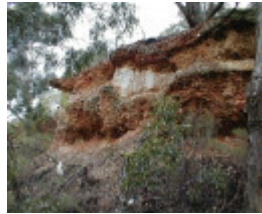
h02047 castlemaine diggings false bottom july02 db
