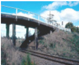
h02054 portland flat road bridge west ele south abutment 0903 mz
