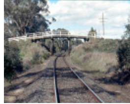
h02054 1 portland flat road bridge west ele 0903 mz
