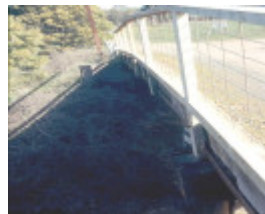
h02054 portland flat road bridge east kerb 0903 mz
