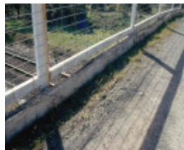
h02054 portland flat road bridge west kerb 0903 mz
