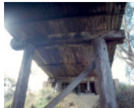
h02054 portland flat road bridge north abutment 0903 mz
