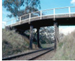
h02054 portland flat road bridge west ele north abutment 0903 mz
