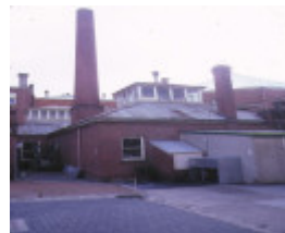
former sandhurst mechanics institute bendigo workshops aug1983
