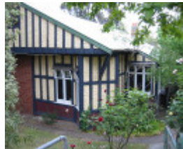
h01033 east view heidelberg front elevation 03 nov2004 mz
