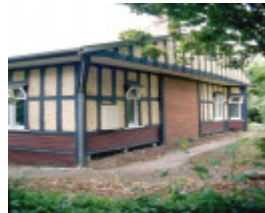
h01033 east view heidelberg front elevation 02 nov2004 mz
