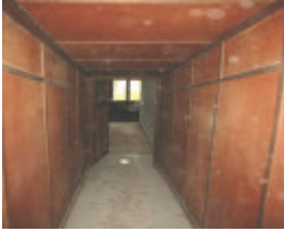
h01033 east view heidleberg tunnel nov2004 mz
