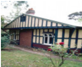
h01033 1 east view heidelberg front elevation 01 nov2004 mz
