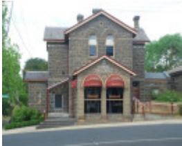
FORMER KILMORE POST OFFICE SOHE 2008
