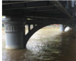
SANDRIDGE RAILWAY LINE BRIDGE October 2016
