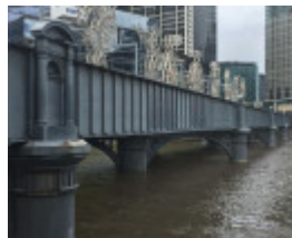
SANDRIDGE RAILWAY LINE BRIDGE October 2016
