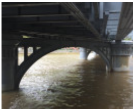
SANDRIDGE RAILWAY LINE BRIDGE October 2016
