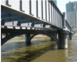
SANDRIDGE RAILWAY LINE BRIDGE SOHE 2008
