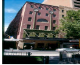
h01542 1 fourth victoria building
