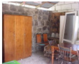
h02071 portland inn bluestone wall 2
