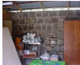
h02071 portland inn bluestone wall
