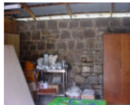
h02071 portland inn bluestone wall
