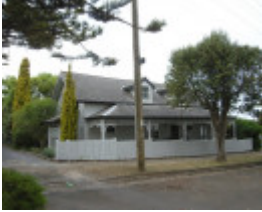
FORMER PORTLAND INN SOHE 2008
