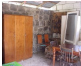
h02071 portland inn bluestone wall 2
