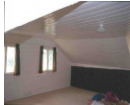
h02071 h2071 former portland inn billiard room july 2004
