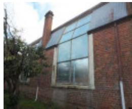
Former Art department, glazing detail, south elevation (Source: CMP, 2021)
