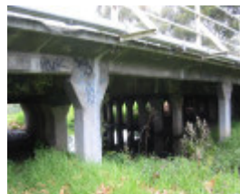
h02080 st kilda street bridge elwood structure west side 03 mz may2005
