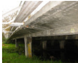
h02080 st kilda street bridge elwood structure west side 01 mz may2005
