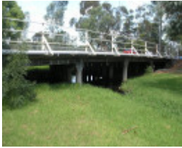
ST KILDA STREET BRIDGE SOHE 2008
