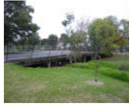
h02080 1 st kilda street bridge elwood east view mz may2005
