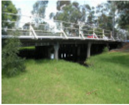
ST KILDA STREET BRIDGE SOHE 2008
