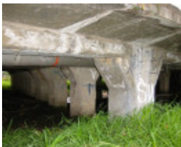
h02080 st kilda street bridge elwood structure east side 01 mz may2005
