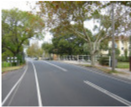
h02080 st kilda street bridge elwood north view mz may2005
