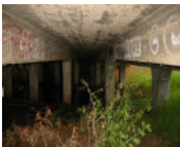
h02080 st kilda street bridge elwood structure west side 02 mz may2005
