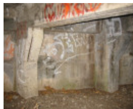
h02080 st kilda street bridge elwood north abutment mz may2005
