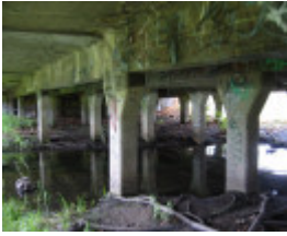
h02080 st kilda street bridge elwood structure under footpath 01 mz may2005
