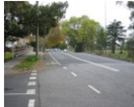
h02080 st kilda street bridge elwood south view mz may2005
