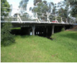
ST KILDA STREET BRIDGE SOHE 2008
