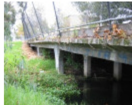
h02080 st kilda street bridge elwood structure east side 02 mz may2005
