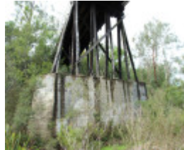
Murrindal truss bridge on cutwater IMG_0939.jpg
