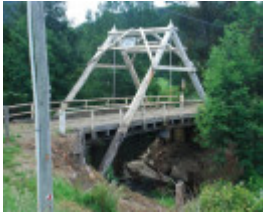
HIAWATHA A FRAME BRIDGE SOHE 2008
