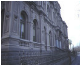
law courts bendigo facade detail jul1984
