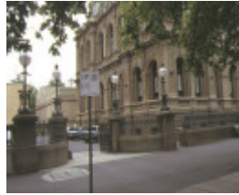
law courts bendigo entrance gates jan1999
