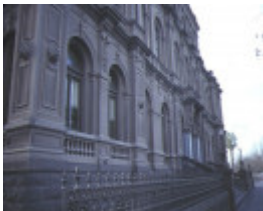
law courts bendigo facade detail jul1984
