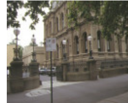
law courts bendigo entrance gates jan1999
