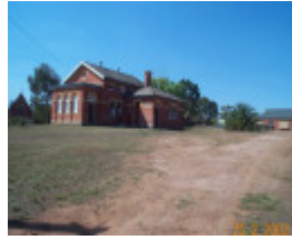
H01120 inglewood court house site degraded histenviro project feb2003
