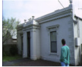
Emoh Cox Street Portv Fairy Front View
