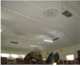
First floor foyer ceiling 2011
