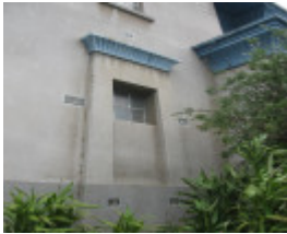
detail of window, front facade 2011
