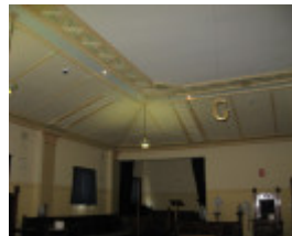
Lodge Room, general view 2011
