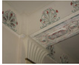
Ground Floor Hall, detail of decoration 2011
