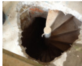
spiral stairway from hub to kitchen below.jpg
