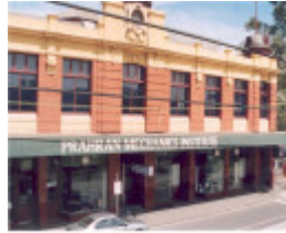
h00400 1 facade full
