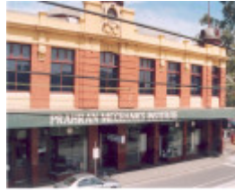
h00400 1 facade full
