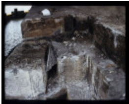
SHEPHERD SWINGBRIDGE ABUTMENT FOUNDATIONS EXCAVATION
