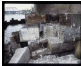
SHEPHERD SWINGBRIDGE ABUTMENT FOUNDATIONS EXCAVATION
