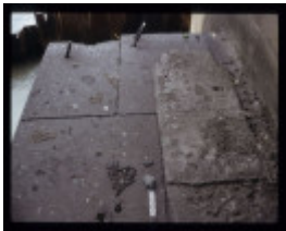
SHEPHERD SWINGBRIDGE ABUTMENT FOUNDATIONS EXCAVATION
