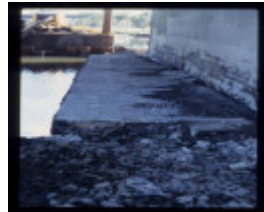
SHEPHERD SWINGBRIDGE ABUTMENT FOUNDATIONS EXCAVATION
