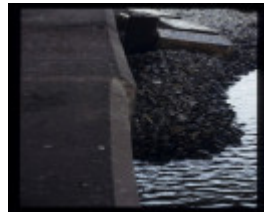
SHEPHERD SWINGBRIDGE ABUTMENT FOUNDATIONS EXCAVATION
