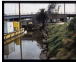
SHEPHERD SWINGBRIDGE ABUTMENT FOUNDATIONS EXCAVATION
