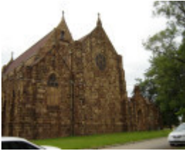
h01065 holy trinity anglican cathedral precinct wangaratta west side 2005
