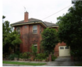
h01065 holy trinity anglican cathedral precinct wangaratta 9 the close 2005
