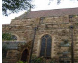
h01065 holy trinity anglican cathedral precinct wangaratta south side 2005
