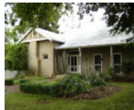
h01065 holy trinity anglican cathedral precinct wangaratta deanery 13 the close 2005
