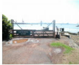
Parson's Boatshed Slipway And Jetty Williamstown March 2003 003
