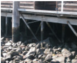
Parson's Boatshed Slipway And Jetty Williamstown March 2003 004
