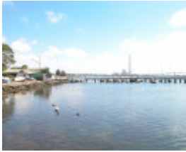
Parson's Boatshed Slipway And Jetty Williamstown March 2003 001
