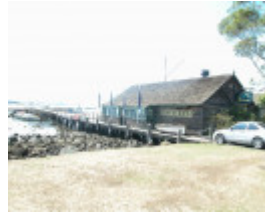
Parson's Boatshed Slipway And Jetty Williamstown March 2003 002
