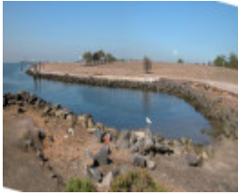
Power Station Park Seawall Williamstown March 2003
