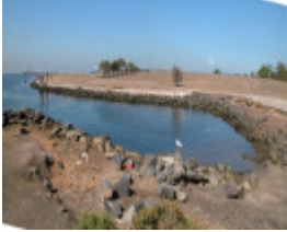
Power Station Park Seawall Williamstown March 2003
