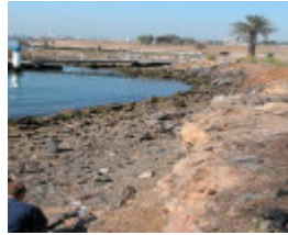
Greenwich Pier Ballast Wharves Piles Williamstown April 2003 001
