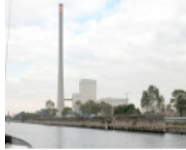
Newport Coal Wharves Williamstown Aug 2003 003
