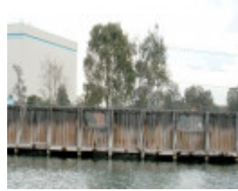
Newport Coal Wharves Williamstown Aug 2003 002
