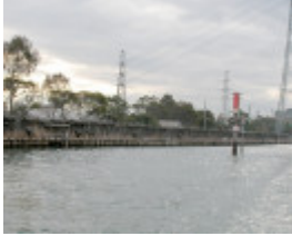
Newport Coal Wharves Williamstown Aug 2003 001
