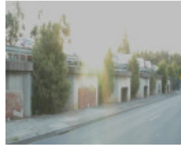
Williamstown Wheat Silos Williamstown June 2003
