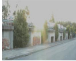
Williamstown Wheat Silos Williamstown June 2003
