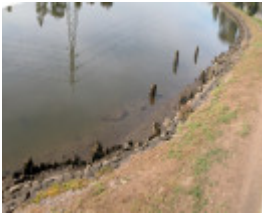
Jack's Magazine Canal And Wharf Maribyrnong July 2003 001
