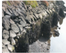
Jack's Magazine Canal And Wharf Maribyrnong July 2003 002
