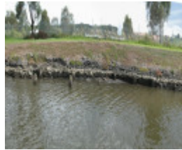
Jack's Magazine Canal And Wharf Maribyrnong July 2003 003
