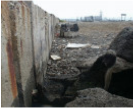
Channel Deepening Project
