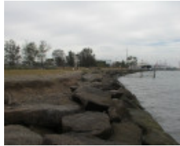
Channel Deepening Project
