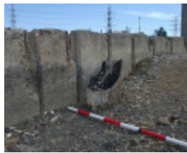
Channel Deepening Project
