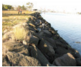
Channel Deepening Project
