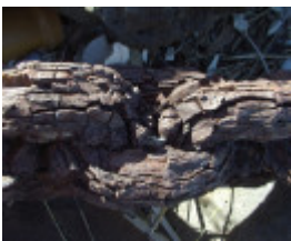
Channel Deepening Project
