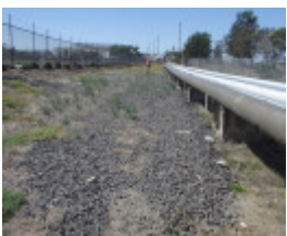
Channel Deepening Project
