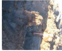
Channel Deepening Project
