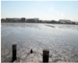
Stony Creek Pier Piles Maribyrnong March 2003 001
