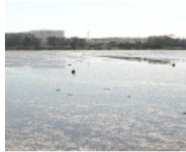
Stony Creek Pier Piles Maribyrnong March 2003 003
