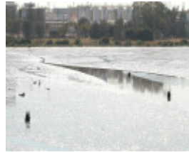
Stony Creek Pier Piles Maribyrnong March 2003 002
