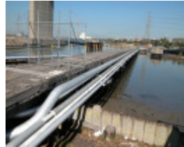
Stony Creek Concrete Sheet Piling Maribyrnong March 2003 002
