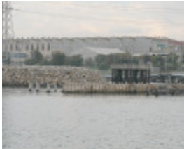
Stony Creek Concrete Sheet Piling Maribyrnong March 2003 001
