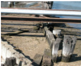
Stony Creek Concrete Sheet Piling Maribyrnong March 2003 004
