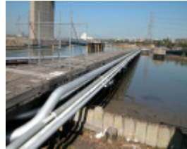
Stony Creek Concrete Sheet Piling Maribyrnong March 2003 002
