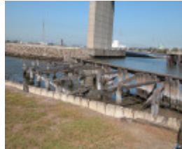
Stony Creek Concrete Sheet Piling Maribyrnong March 2003 003
