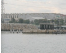
Stony Creek Concrete Sheet Piling Maribyrnong March 2003 001
