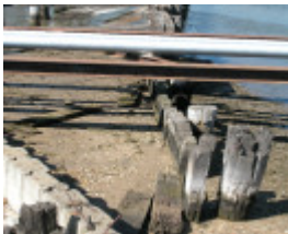
Stony Creek Concrete Sheet Piling Maribyrnong March 2003 004
