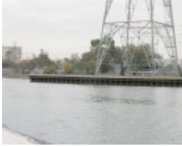
Newport Oil Wharves Williamstown June 2003 001
