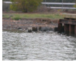
Newport Oil Wharves Williamstown June 2003 002
