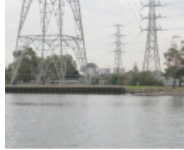
Newport Oil Wharves Williamstown June 2003 003
