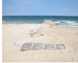
Harold St Drain Port Melbourne April 2006 003
