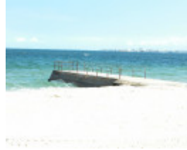
Harold St Drain Port Melbourne April 2006 002
