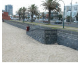
Albert Park Baths Site March 2003 Embankment Stairs 003
