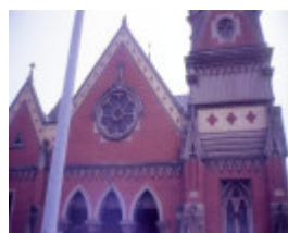
former congregational church and hall mair and dawson sts north ballarat windows she project 2004
