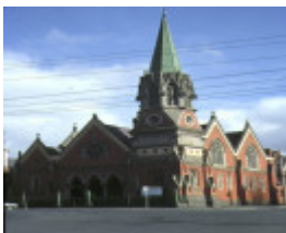
1 former congregational church ballarat front view aug1985
