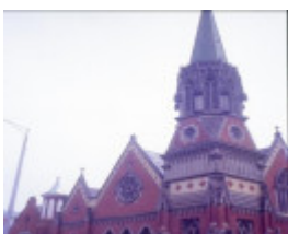
former congregational church and hall mair and dawson sts north ballarat steeple she project 2004
