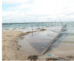
Lagoon Training Walls Wharves And Drain Port Melbourne April 2003 Groyne And Drain 003
