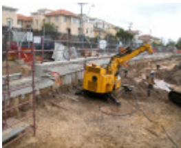
Lagoon Training Walls Wharves And Drain Port Melbourne April 2003 Construction Site 004
