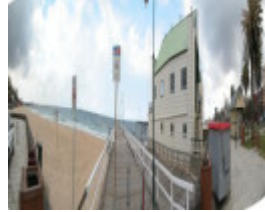
Kerferd Road Pier Port Melbourne March 2003 002
