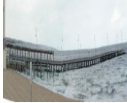
Kerferd Road Pier Port Melbourne March 2003 003
