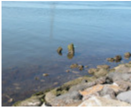
Spotswood Pumping Station Wharf Piles Williamstown May 2003
