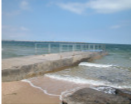
McGregor Street Drain Culvert Port Melbourne March 2003
