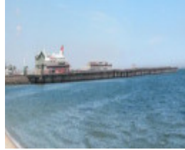
Princes Pier Port Melbourne March 2003 001
