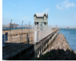
Princes Pier Port Melbourne March 2003 003
