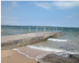
McGregor St Unidentified Stone Structure Port Melbourne March 2003 McGregor St Drain 001
