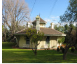
Flemington racecourse_former Convalescent jockeys Lodge_KJ_July 09 July 09
